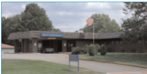
Riverview Rehabilitation Center 1041 Hill Street, Wisconsin Rapids
